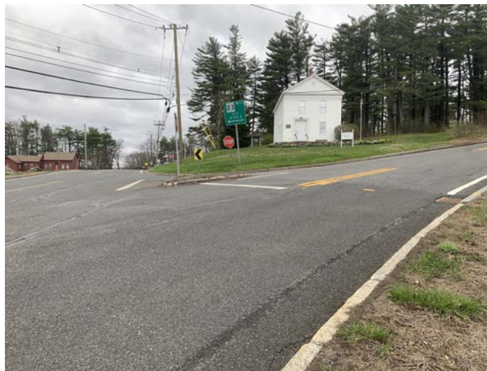
Existing North Street/Rt. 23 intersection has no marked crosswalk. A reconfiguration of the intersection could provide a protected crossing for people walking from the parking area to the Historical Society building.
